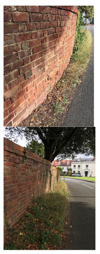
The verge has been eroded from approximately 1m to 15cm wide by vehicles having to drive very close to the brick wall to avoid oncoming vehicles. There are chips and gouges from impacts seen on the brickwork.
